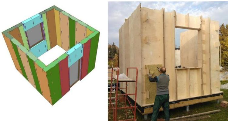
Fig. 4 Plywood frame structure installation design (type C)
